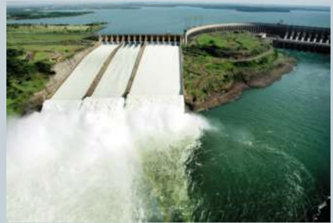
Itaipu Dam in Parana River → supply electricity in Brazil & Paraguay
